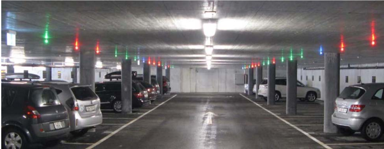
Figure 5.9 - Single-space guidance parking system installed at Colorado State University.
