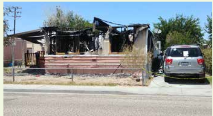
House burned down in Ridgecrest Quake, photo by Syd Kotar
