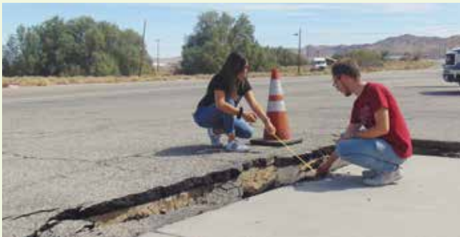
Syd Kotar '19 and Muhammad Karkoutli '20 measure a crack created by the Ridgecrest Quake
