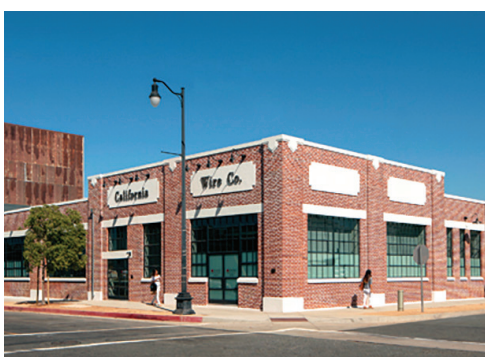
Among the elements of the building renewal was the restoration of its original brick façade.
