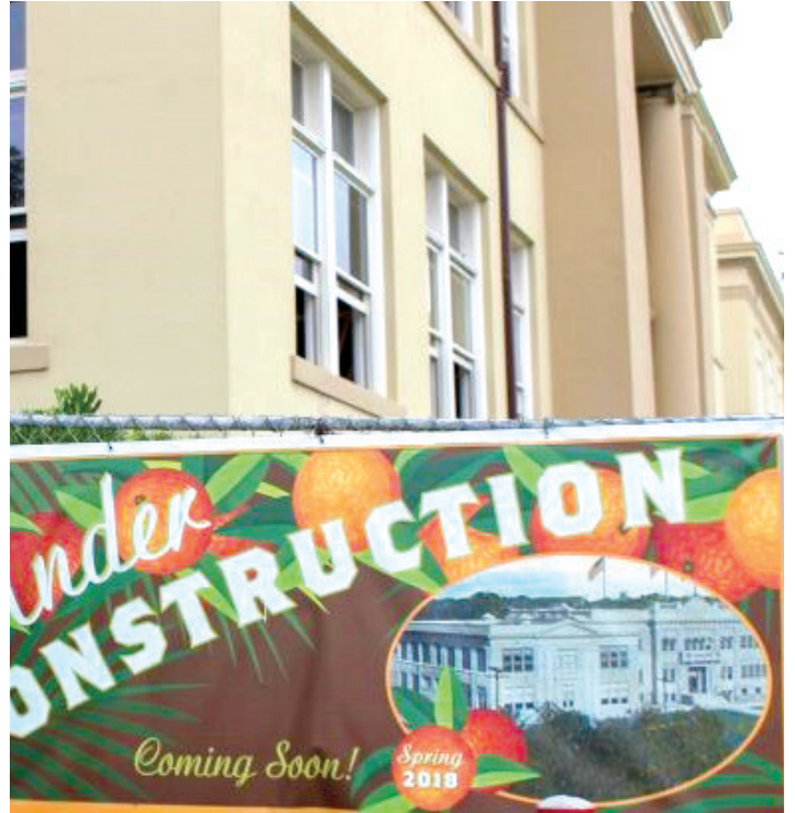
Historic Reeves Hall will retain its historic character when safety and modernization upgrades are complete. (Photo/Amanda Glemmo '20)
