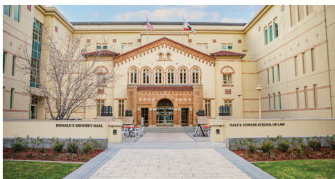
Converting to drip irrigation at Kennedy Hall resulted in annual savings of more than 180,000 gallons of water.
